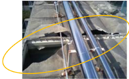
(b) On-ground FRP tank (Sendai, 1988)
