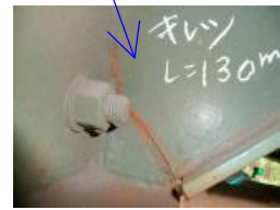
図-4 槽状桁端支材のき裂
