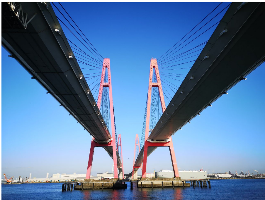
Figure 1 Meiko Nishi Bridge (completed in 1985 and 1997), Nagoya, Japan
