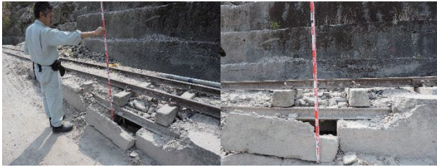
Figure 13 Raised Railway Track of DHR (H=20cm)
