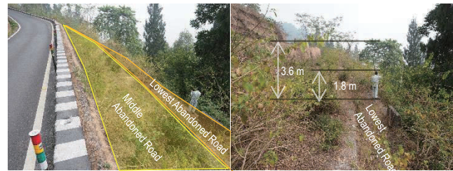
Figure 16 Abandoned Road of NH55 at RS4
