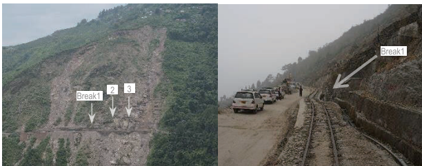
Figure 8 Deep-seated Landslide (Left) and Bending and Sinking of Highway and Railway Track (Right) in 2017 2)
