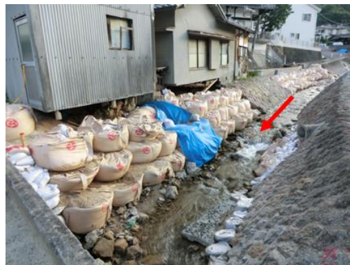
(c) 地点⑤での護岸の破壊
