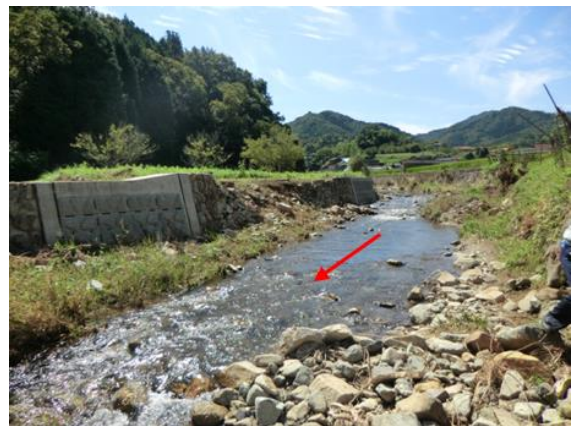
(c) 地点⑥での護岸の破壊
