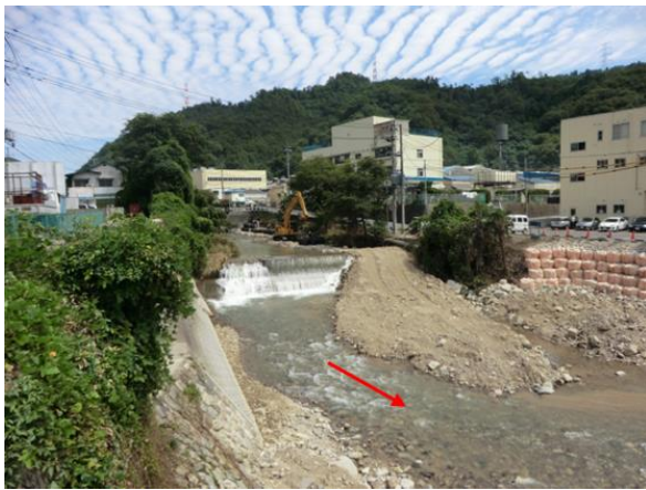
(c) 堰の下流部：護岸の破壊と側岸浸食
