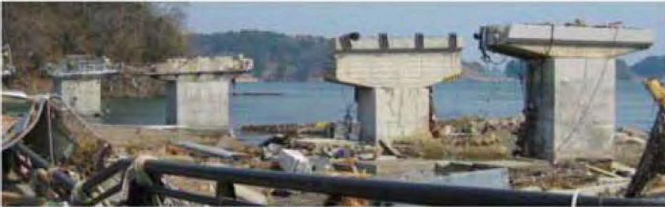
(a) The substructures were left sound
