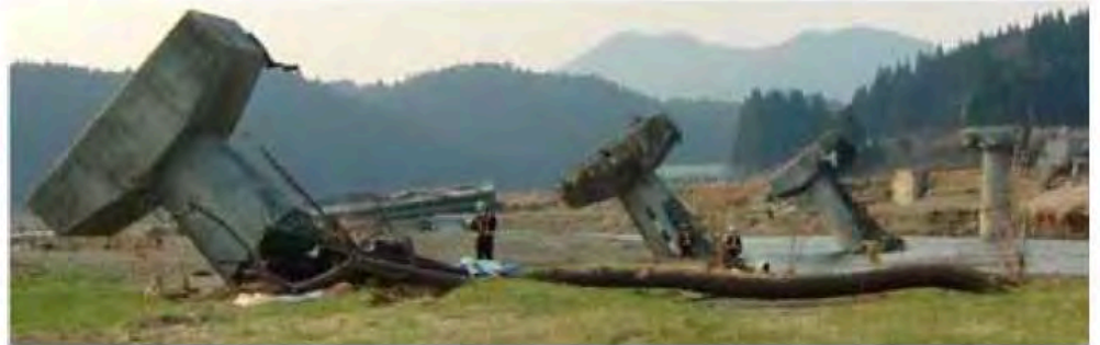
(b) The substructures were pulled down
