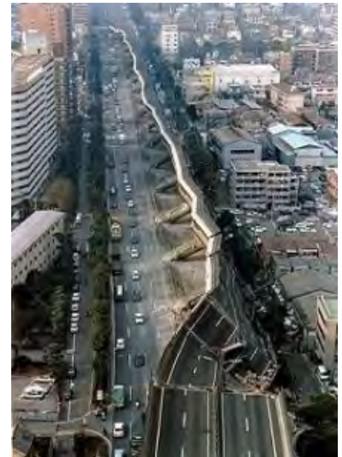
Collapse of Highway (Kobe EQ)
