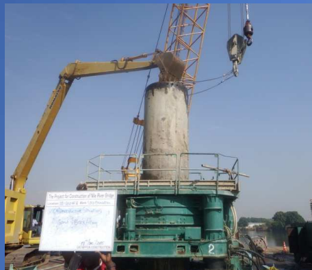
掘削孔の砂充填状況
