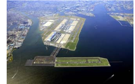
Haneda D-Runway in 2010 ©Kanto Regional Development Bureau, MLIT
