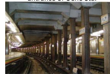
Ginza Line running between Ueno & Ginza 協会50周年記念事業 鉄道施設50選 ©Japan Railway Civil Engineering Association
