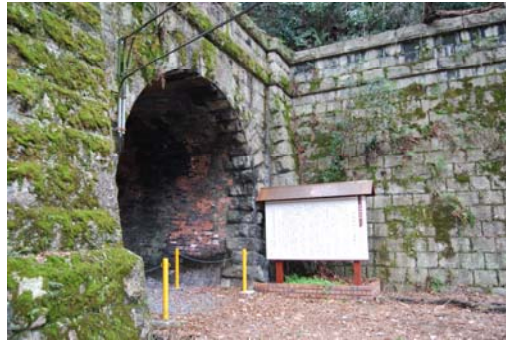
Old Osakayama Tunnel on Tokaido Main Line
