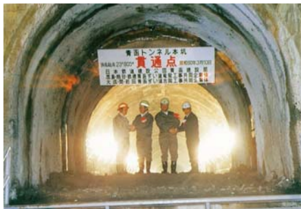
Main tunnel breakthrough ceremony
