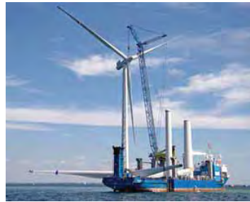
Leg-stabilised crane vessel A2Sea Sea Power
