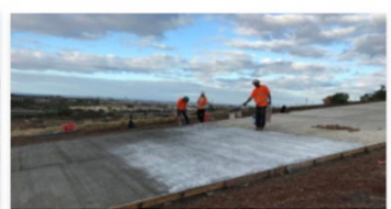
Kapolei Interchange Phase II Honolulu, HI Island Ready-Mix CO 2 Saved: 1,500 LBS / 680 KG
