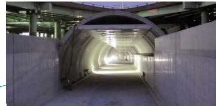
Oi District Tunnel on Shinagawa Line of the Central Circular Route
