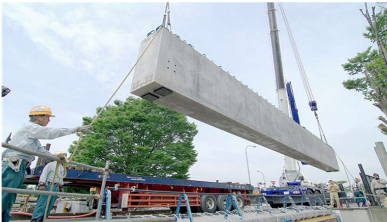
Erecting prestressed concrete girder
