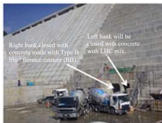
Casting LHC in Apporo Dam Closure Work
