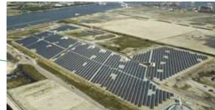
Mega solar power plant "Hikarinomori" on Yumeshima Island, Osaka
