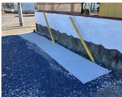
Photo 20.5 Concrete slab on grade
