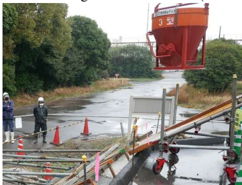
Photo 20.3 Slope protection concrete
