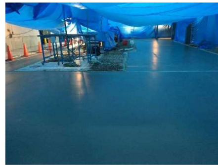
After finishing low-carbon concrete
