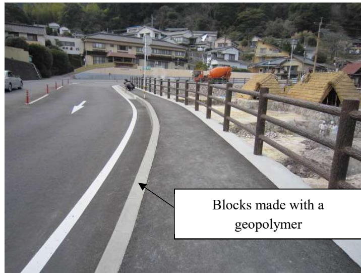
Photo 19.1 Installation example
