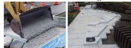
Cast-in-place concrete pavement work
