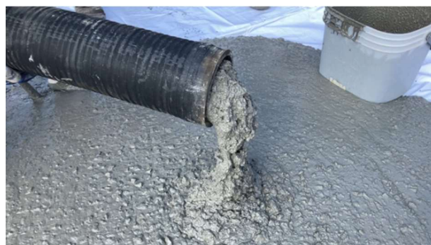
Situation of PolymerCrete discharged through a pipe after pumping
