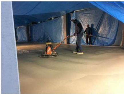
Finishing low-carbon concrete
