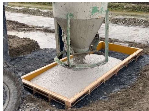
Photo 20.2 Confirmation of fluidity and filling properties on earthen floor
