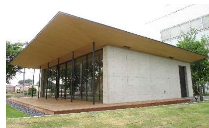
Combination of Clean-Crete and clear paint for the external wall of a facility in the Technical Research Institute of Obayashi Corporation
