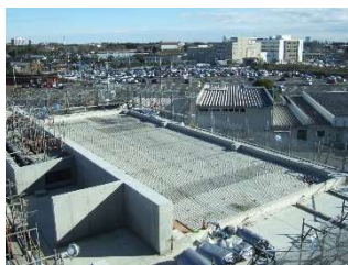
Photo 26.1 Green Office Building
