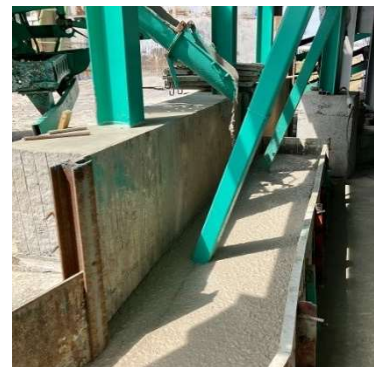
Photo 20.4 Reinforcing building foundation (additional cast-in-place concrete)
