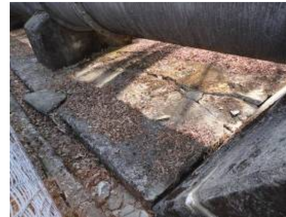
⑤水圧管路敷亀裂
