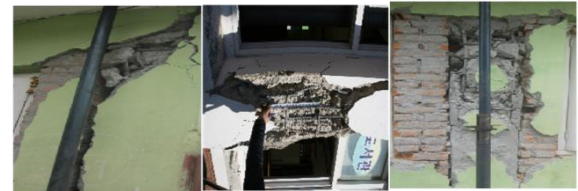
Column Damage Lv2
