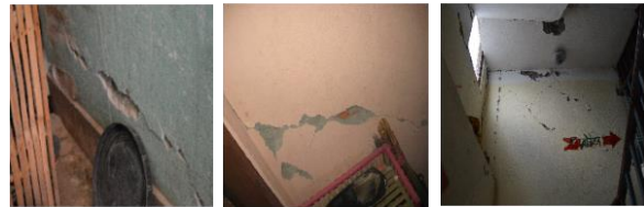
Infill_Wall_Damage Lv1
