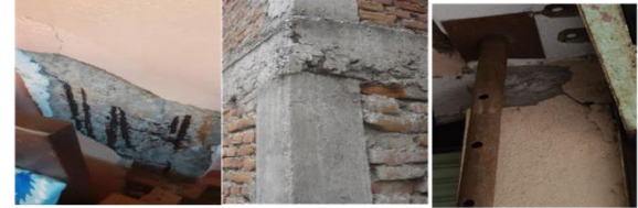
Column Damage Lv2
