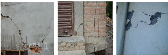
Infill_Wall_Damage Lv3
