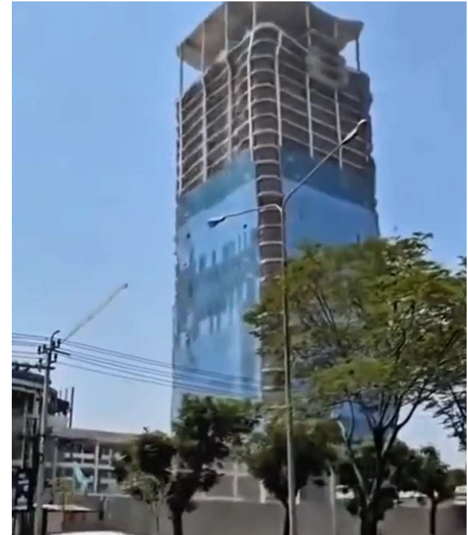
Collapsing 30 floor high-rise building in Bangkok
