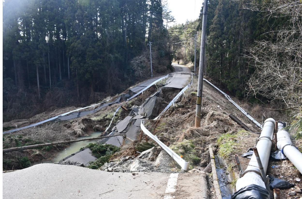
Collapse of road embankment (Map②)
