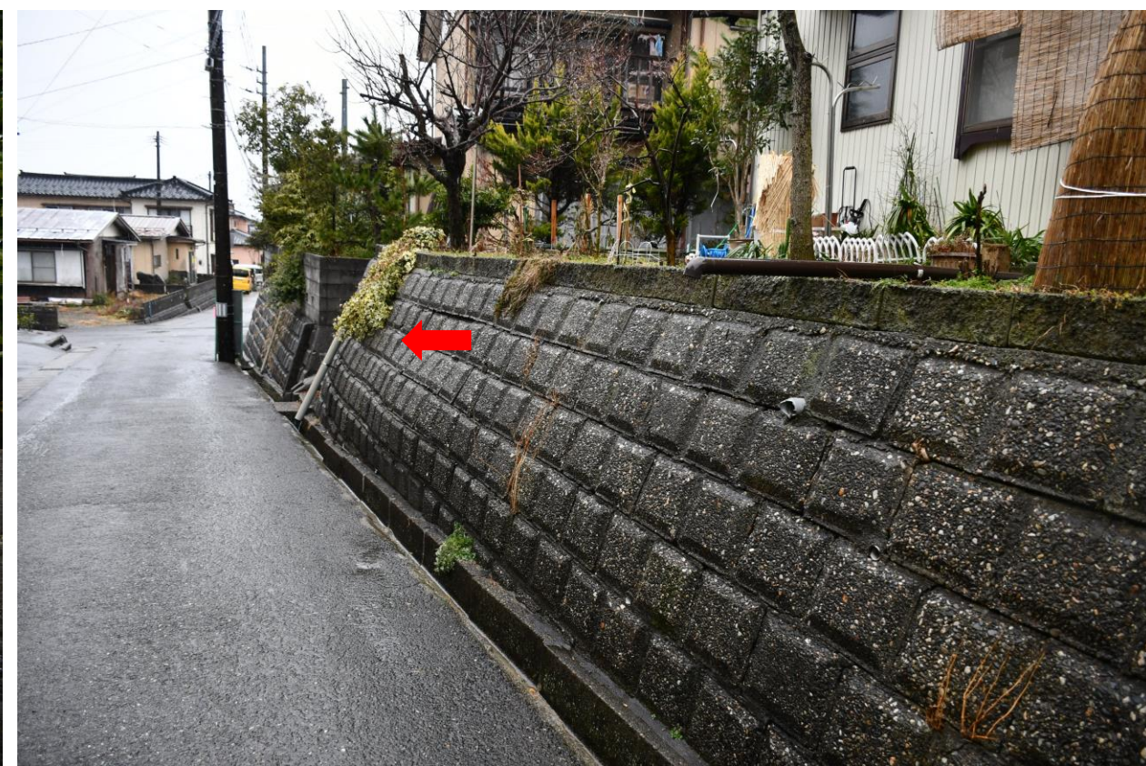
Overhanging of retaining wall (Map①)
