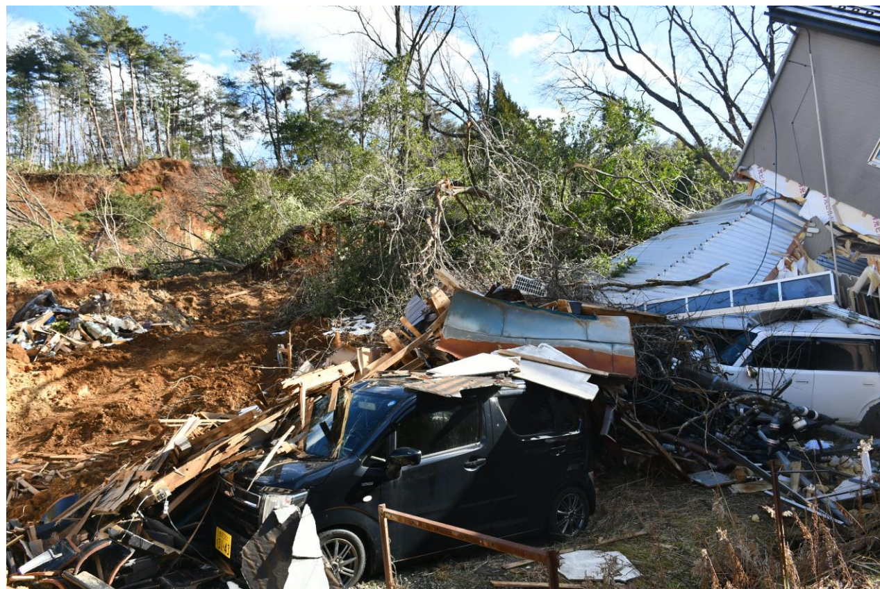
Collapse of wooden house by landslide (Map ①)
