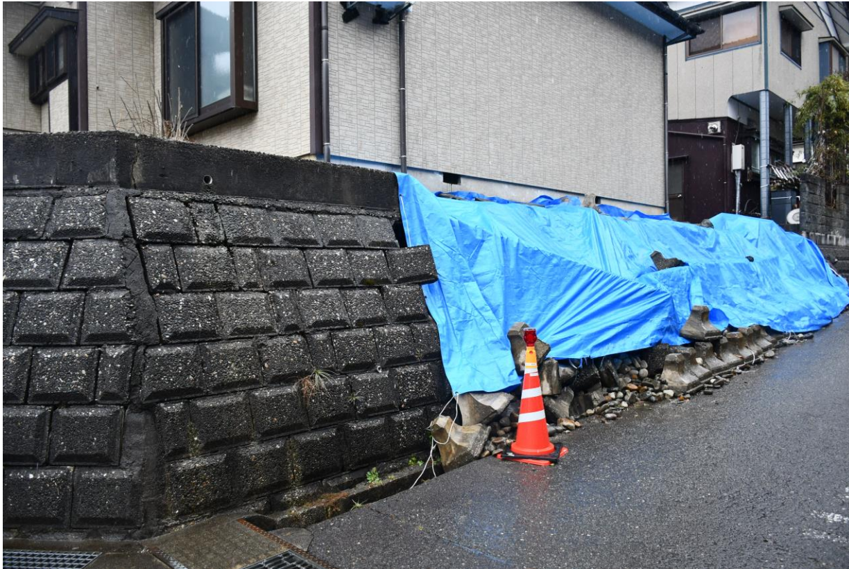
Collapse of retaining wall (Map①)
