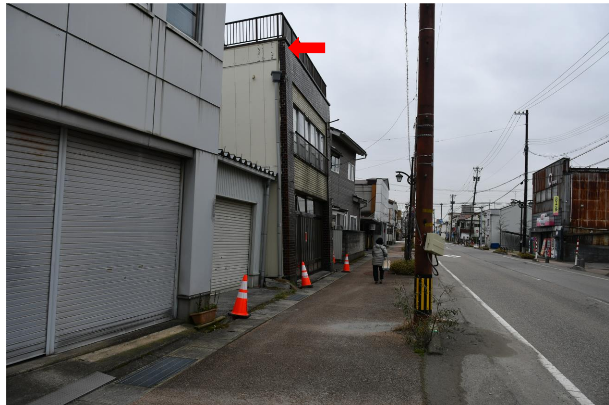
Subsidence and tilting of houses due to liquefaction on flat ground (Map①)
