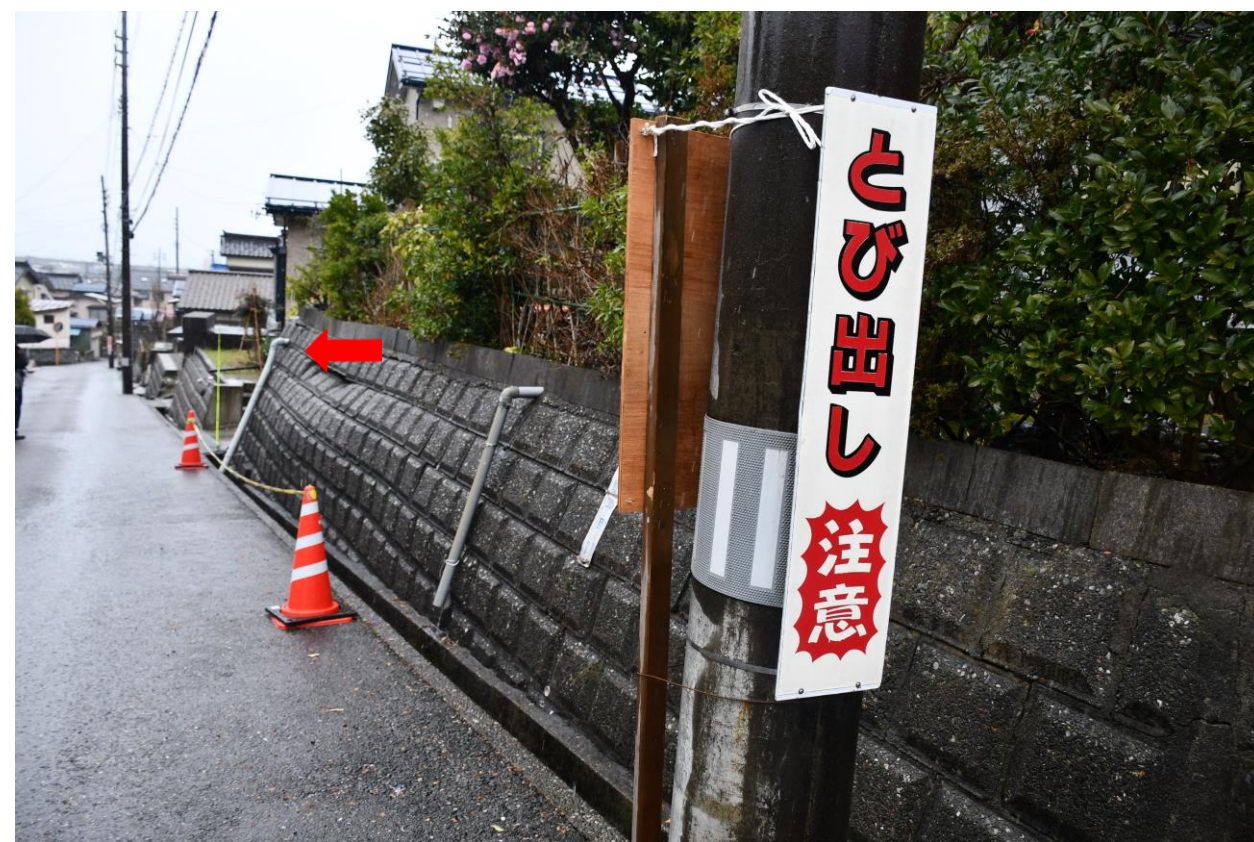
Overhanging of retaining wall (Map①)
