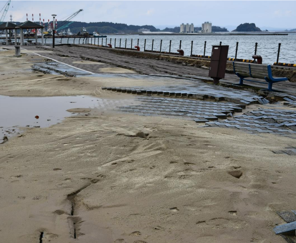
Subsidence and ejected sand due to liquefaction (Map④)
