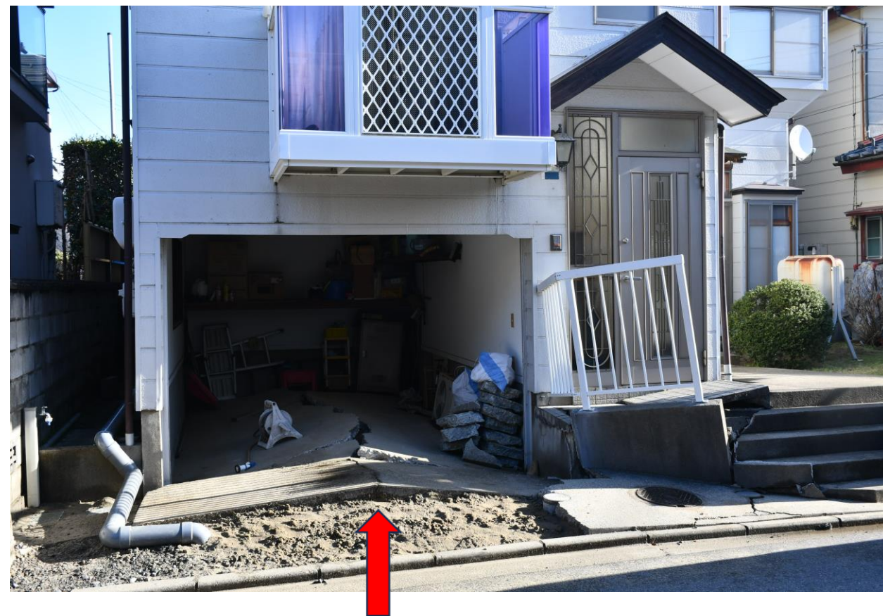
Uplift of the ground due to lateral flow (Map①)
