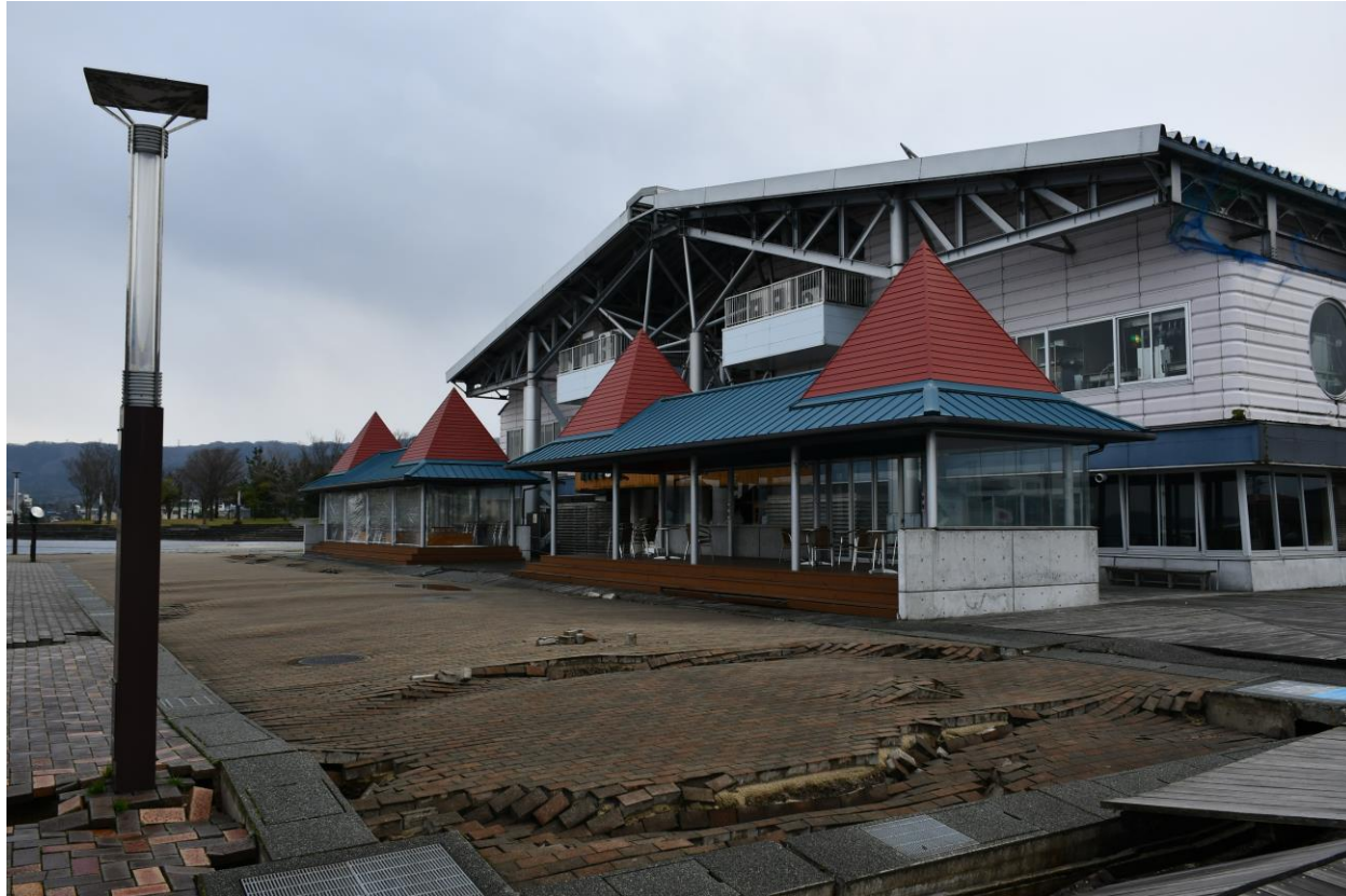
Damage of “ Food Festival Market” induced by liquefaction (Map④)
