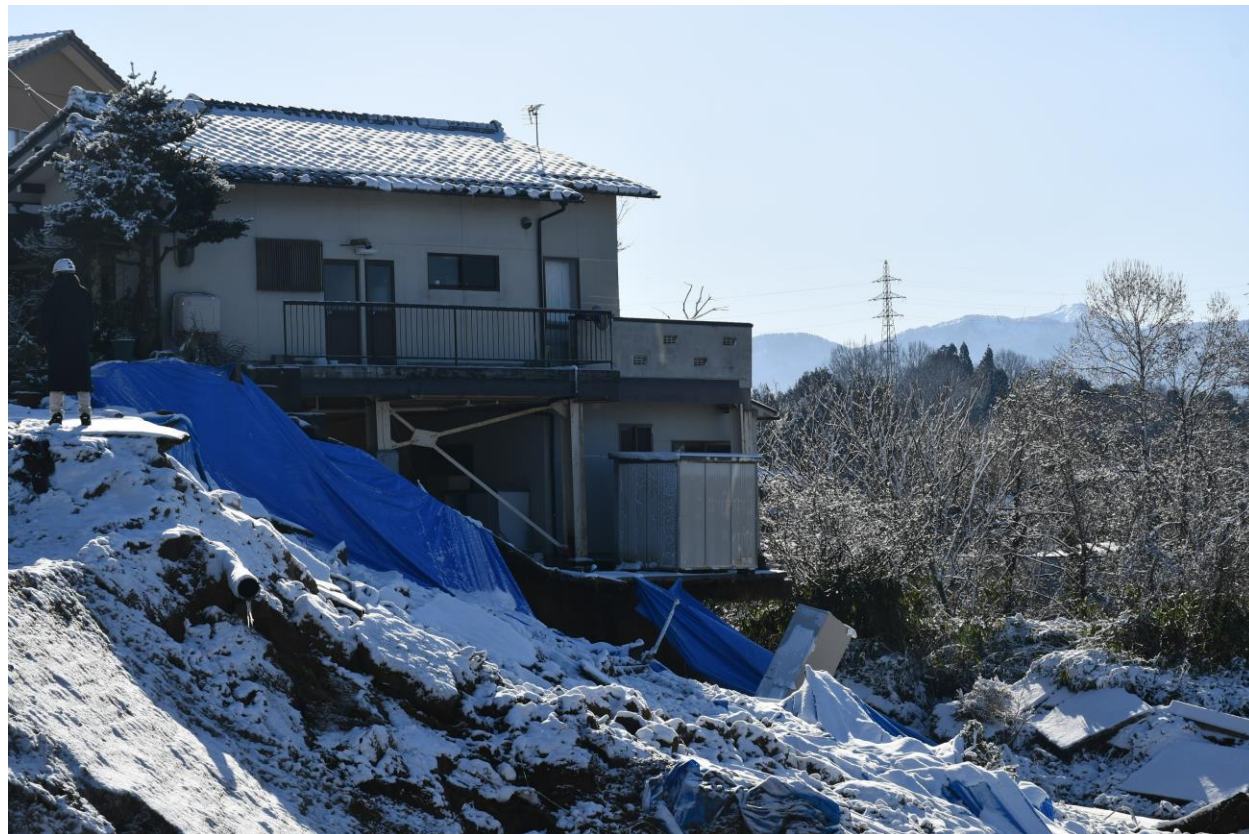
Damage to houses caused by landslides on embankment of developed residential areas (Map①)
