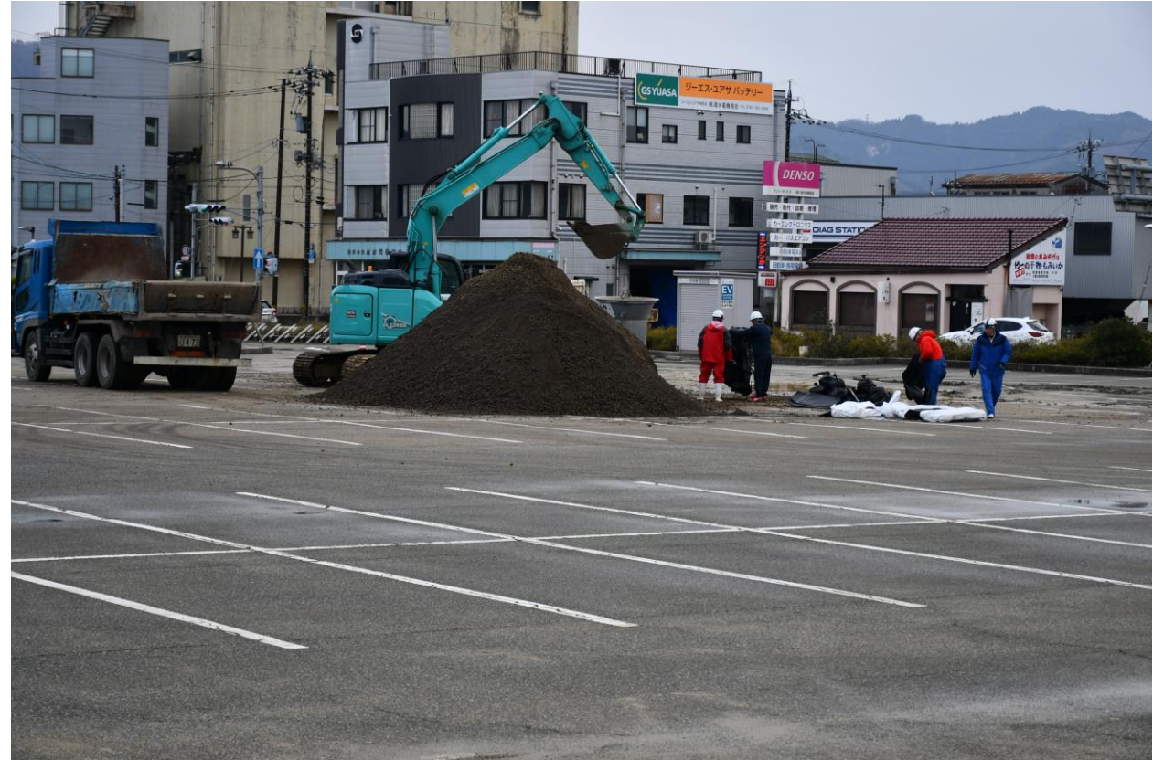
Removal of a large amount of ejected sand in the parking lot (Map④)
