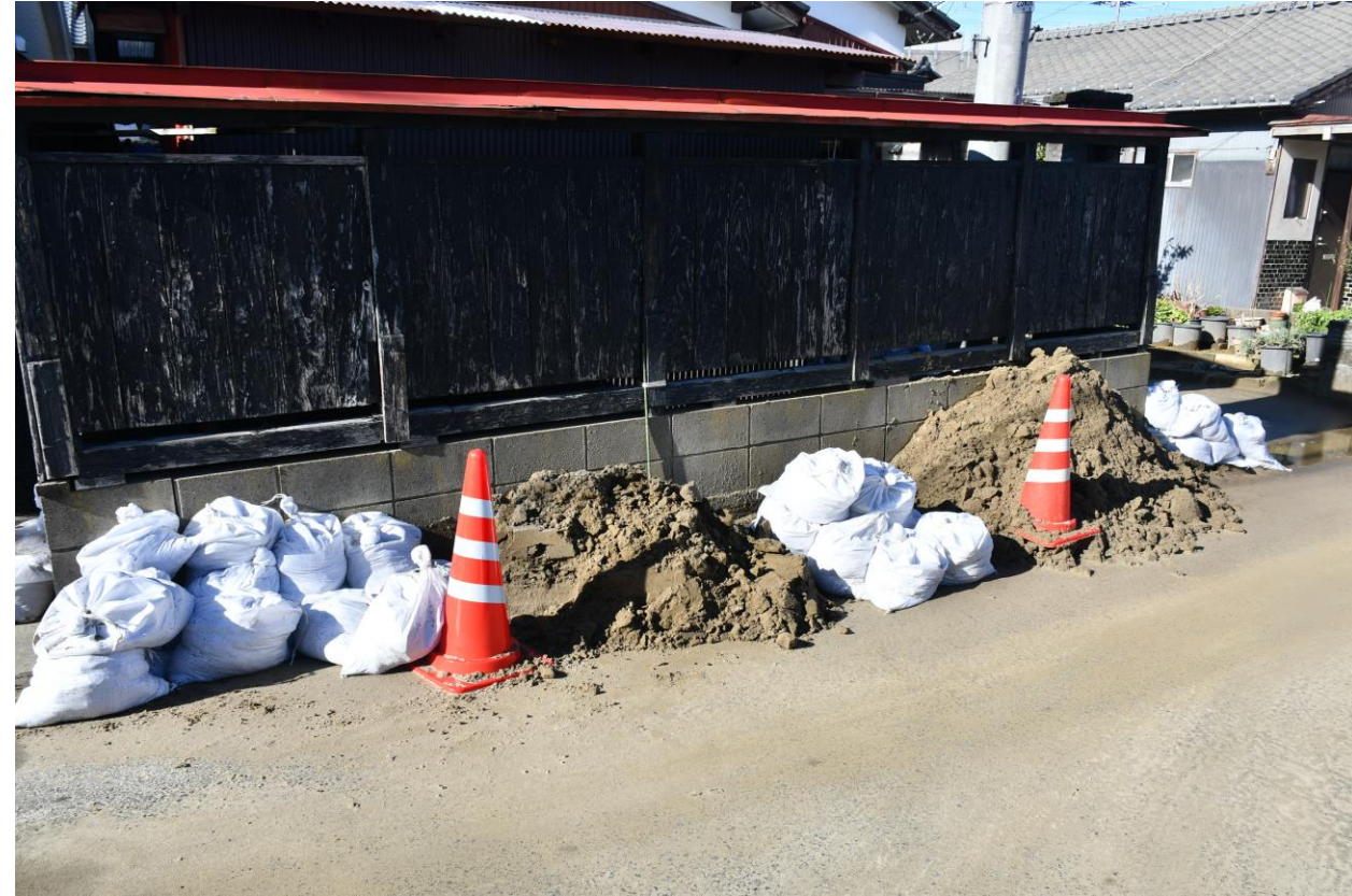
Inclination of houses and large amounts of ejected sand due to liquefaction on flat ground (Map②)
