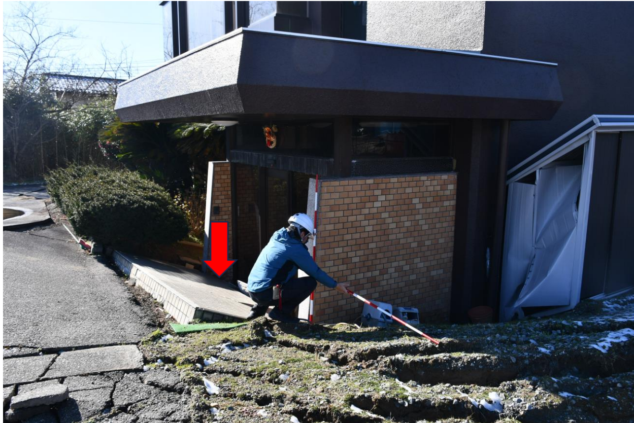
Subsidence of RC building due to liquefaction (Map②)
