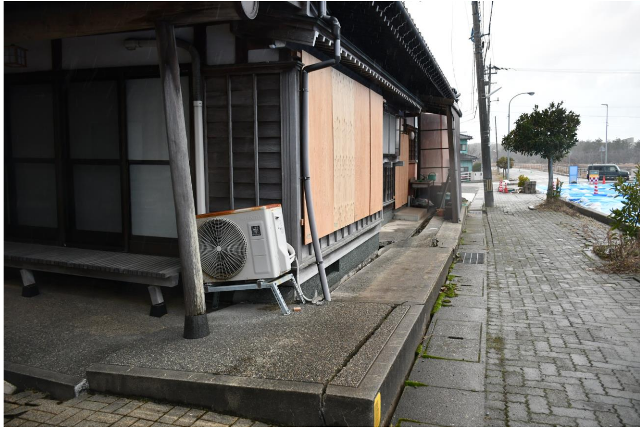
Subsidence and inclination of houses due to liquefaction (Map①)
