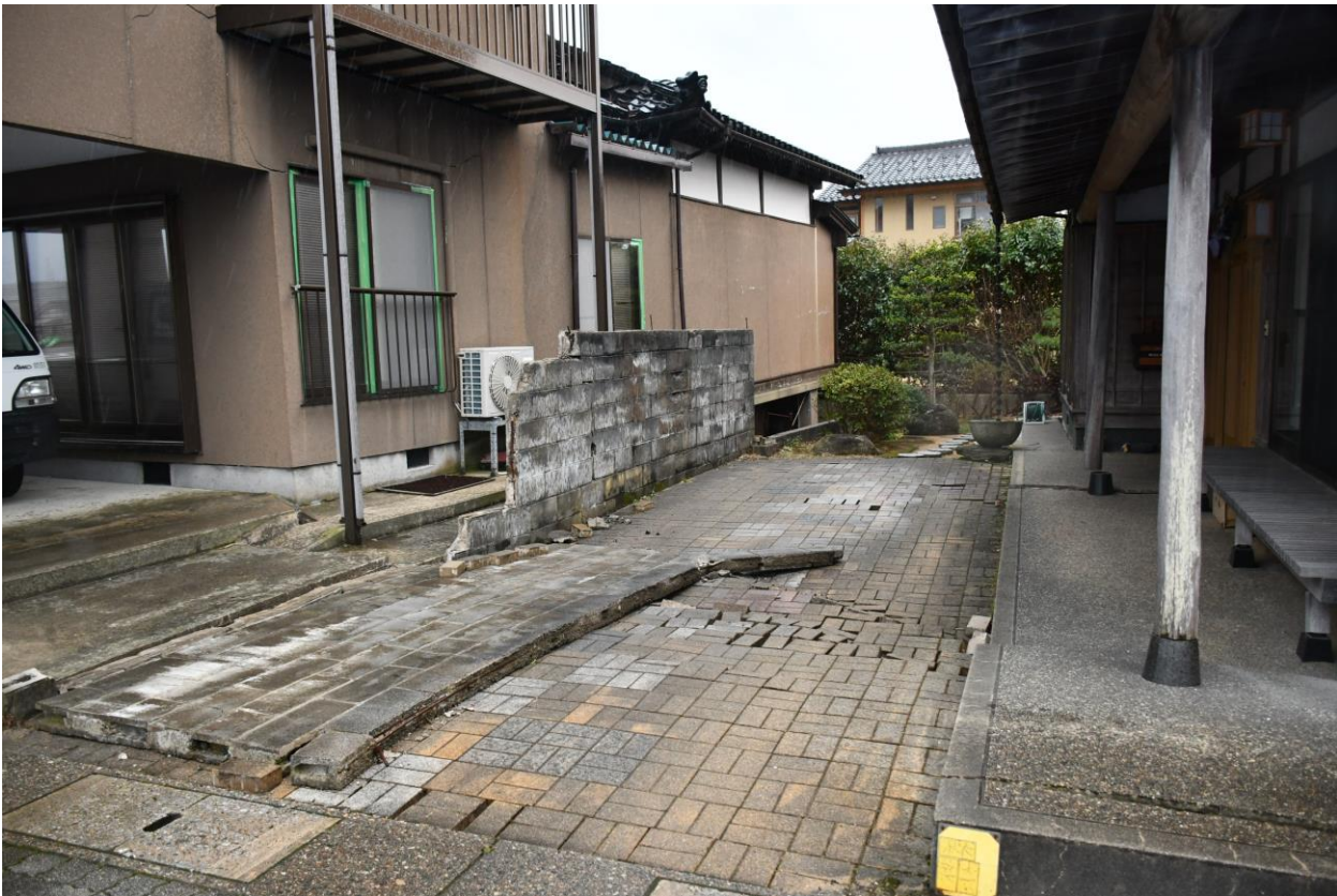
Subsidence and inclination of houses due to liquefaction (Map①)
