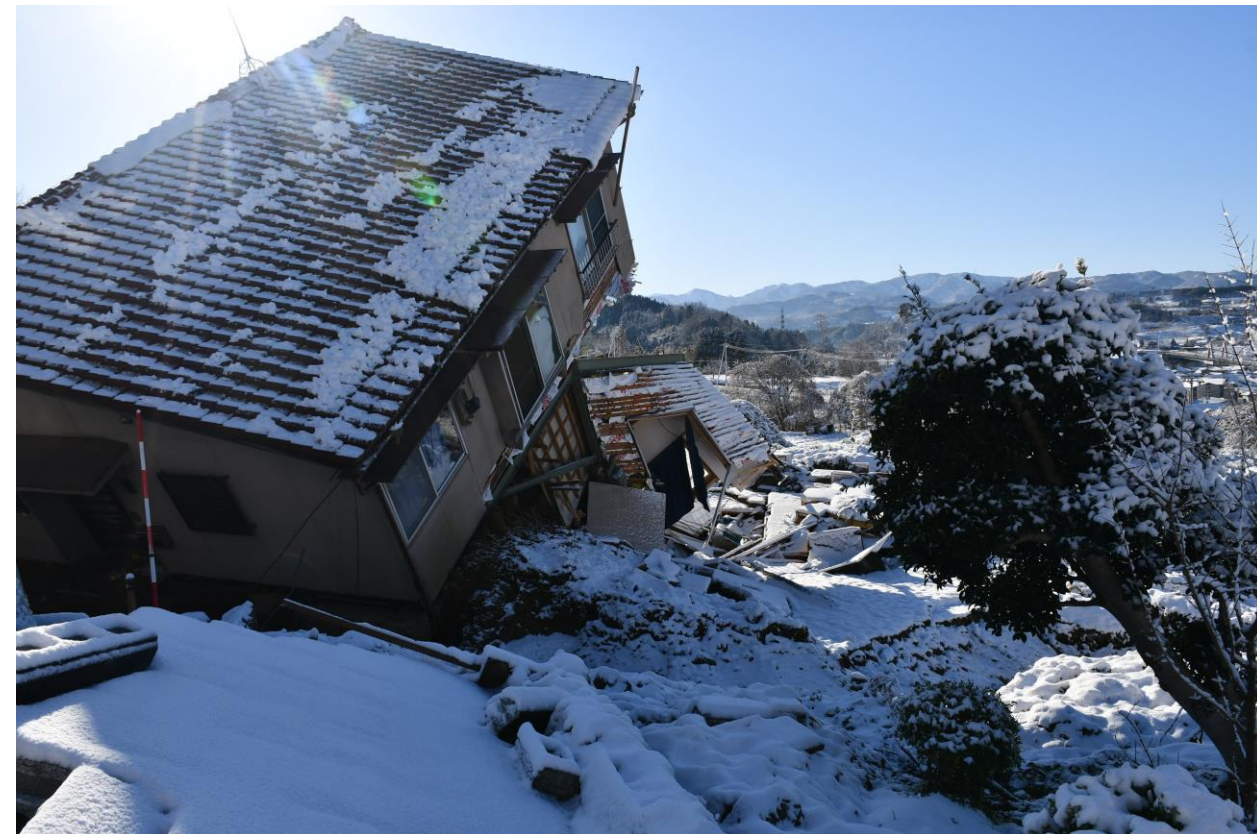
Damage to houses caused by landslides on embankment of developed residential areas (Map①)
