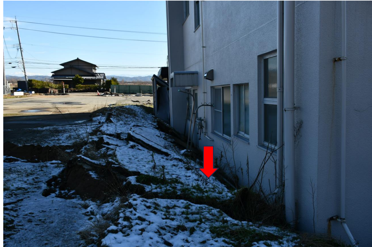
Subsidence of RC building due to liquefaction (Map②)
