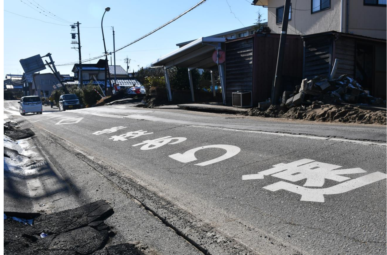
Meandering of the road due to lateral flow of liquefied ground (Map③)
