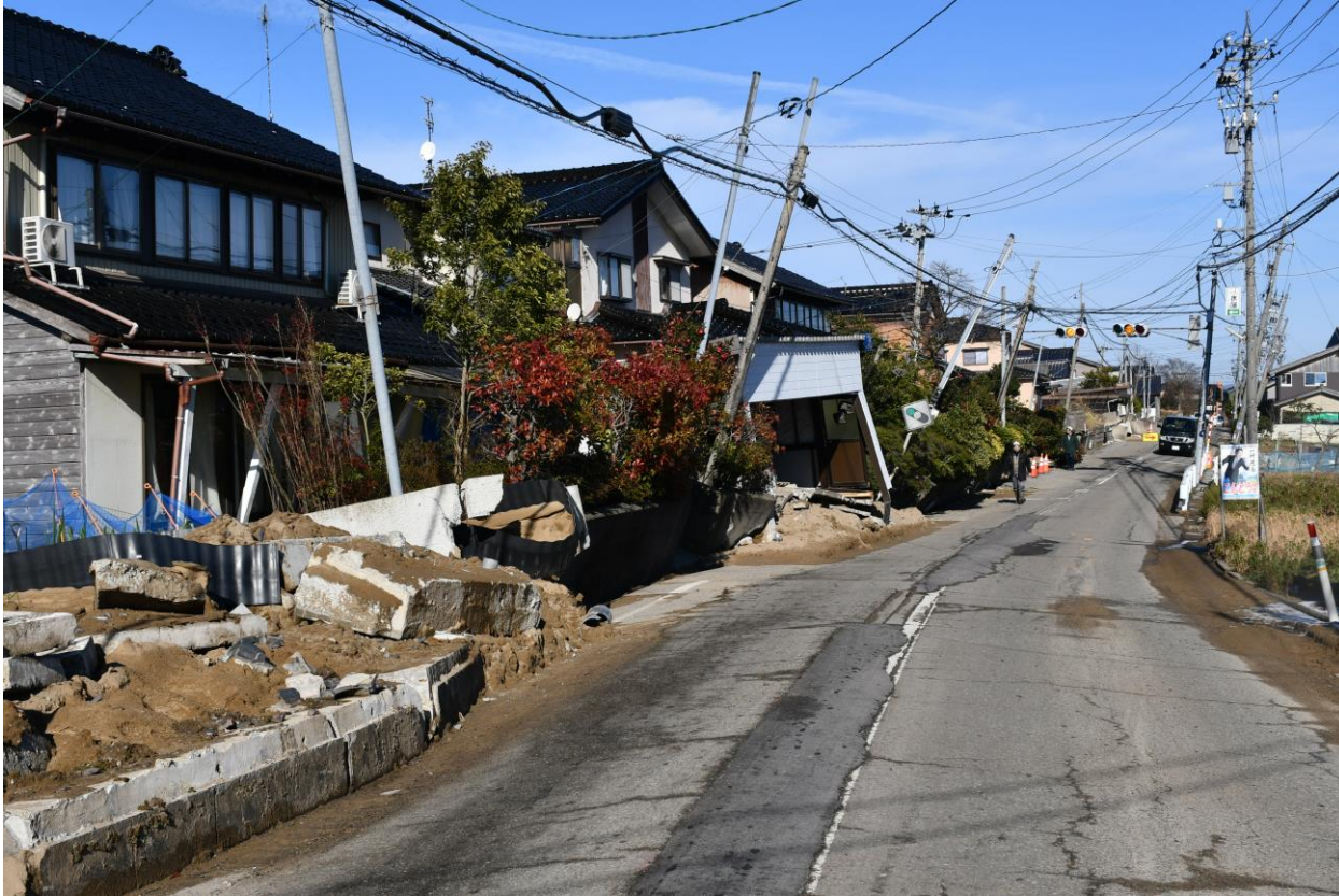
Meandering of the road due to lateral flow of liquefied ground (Map③)
