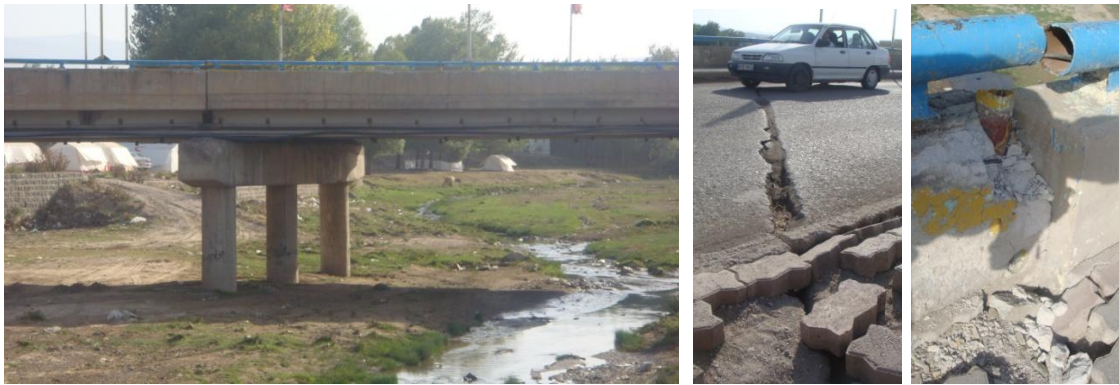
Photo 7 Damage to 6-span composite bridge (No.2)
