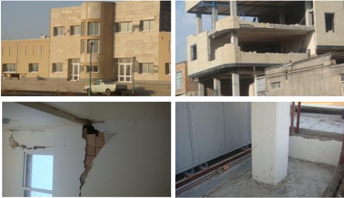
Photo 4 Damage to reinforced concrete buildings
