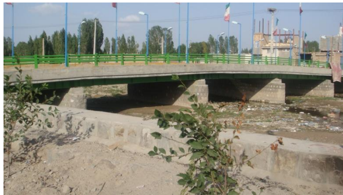
Photo 8 3-span integral composite bridge (No.3)
