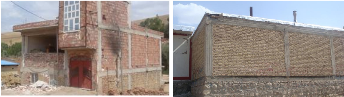
Photo 3 Damage to half reinforced masonry buildings
