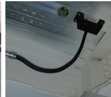
TA on ceiling
