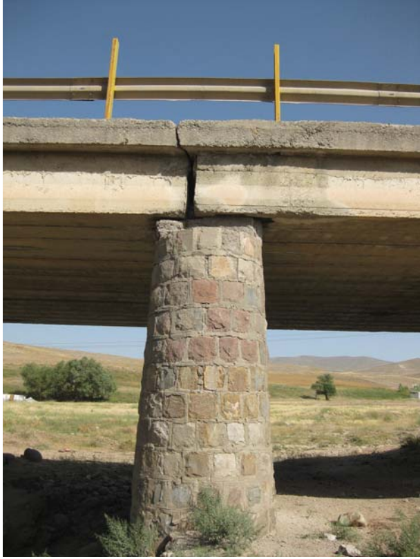
Sliding of the bridge- West View
