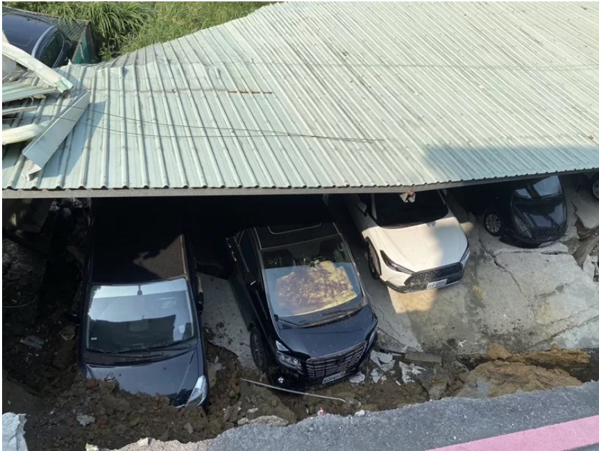
Seven buildings sinking
