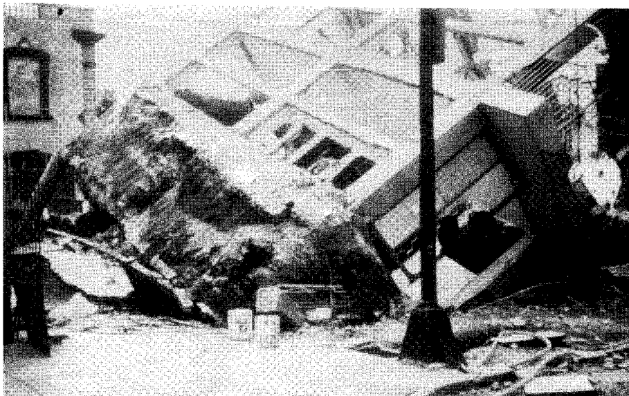
Figure 12 - View of collapsed Building V.
