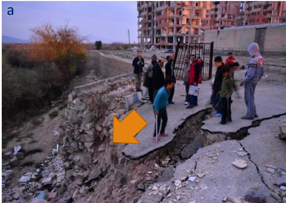
Fig. 10(a and b) Ground deformation in Maskane Mehr/Fooladi District
