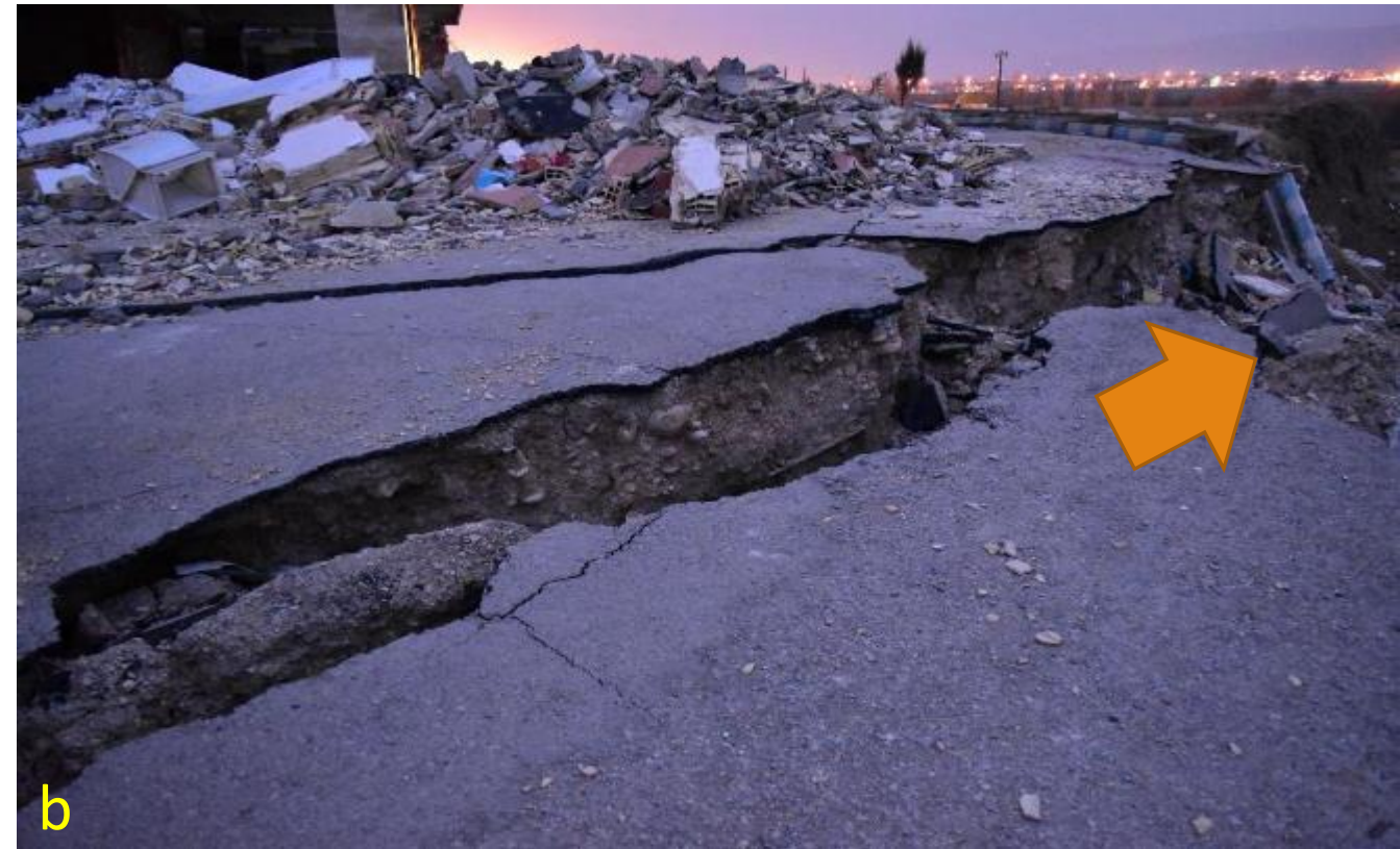
Fig. 10(a and b) Ground deformation in Maskane Mehr/Fooladi District
