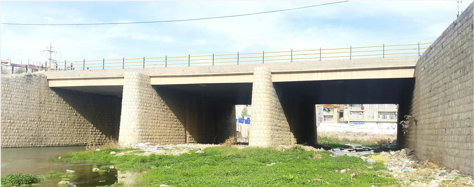
Main bridge of Sarpole-Zahab city
