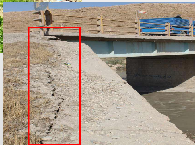
Bridge on road of Sarpole-Zahab to Tazeh-Abad
