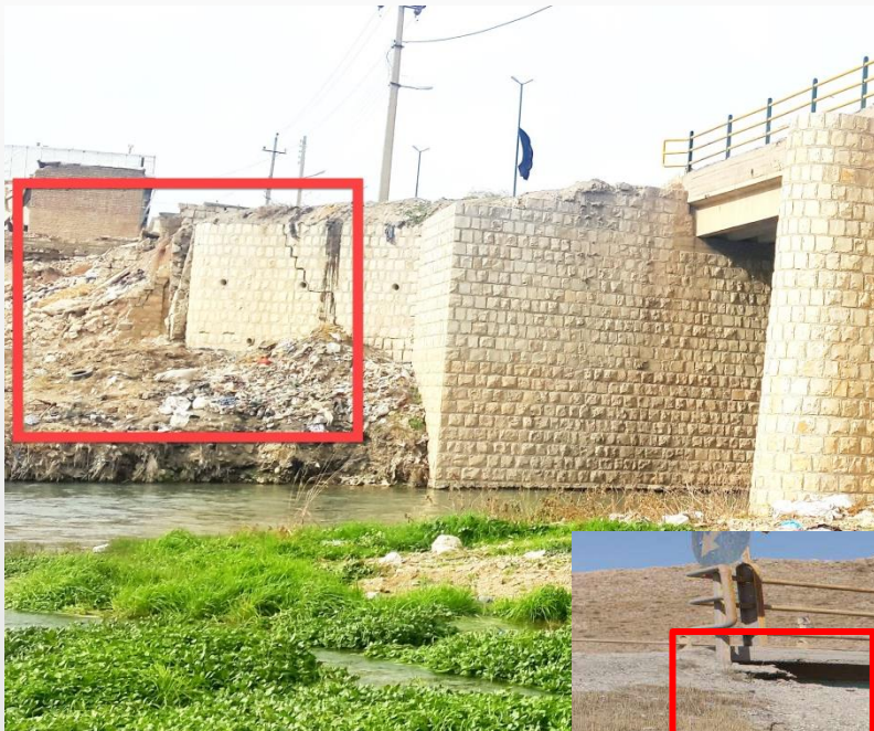
Main bridge of Sarpole-Zahab city
