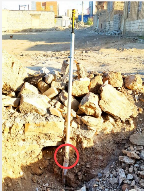
Damage to joint of the gas pipeline at the entrance to the houses at Ahmad-Abad town of Sarpole-Zahab city.
