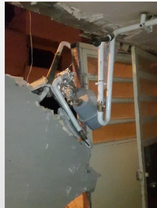
Damage to joint of the gas pipeline at the entrance to the houses at Ahmad-Abad town of Sarpole-Zahab city.
