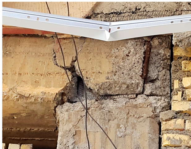
(b) Short anchorage length at rebar of the beams.
