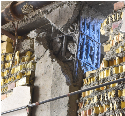
(a) Wide spacing between transverse rebar of columns
