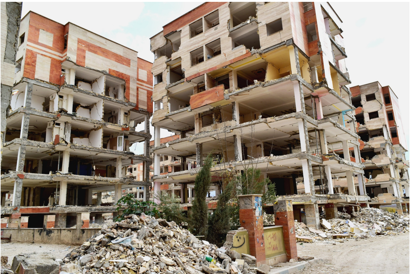
Severe non-structural elements damage at Maskane-Mehr of Sarpole-Zahab city.
