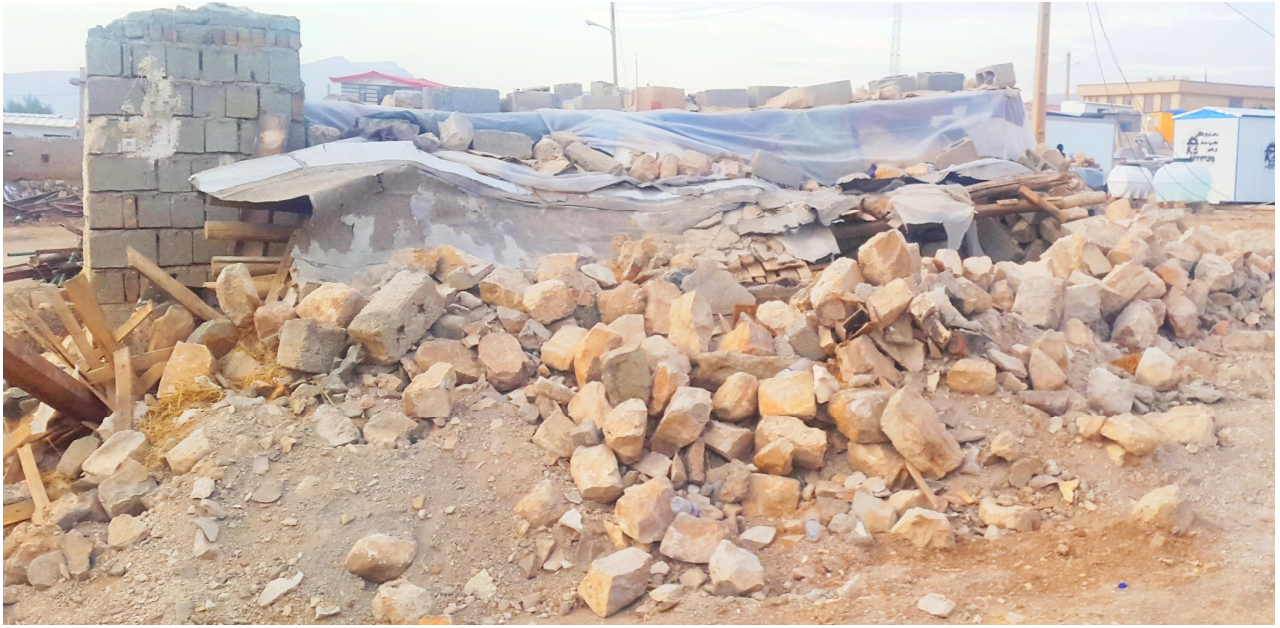
Failure of most of stone buildings in Kuik Village.
