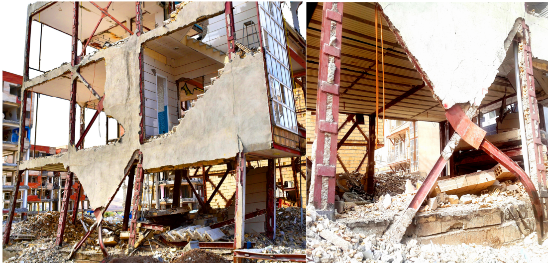
Severe damage to a steel building at Sarpole-Zahab city.
