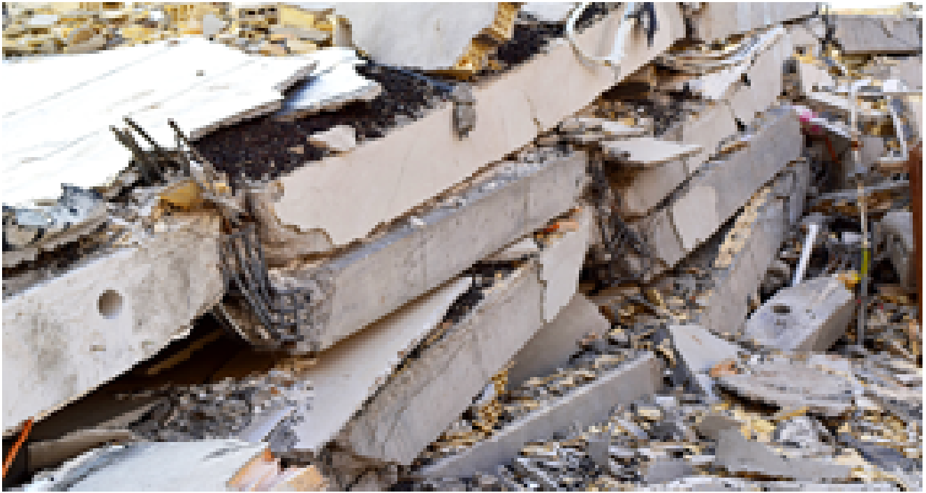
Soft story failure at Sarpole-Zahab city.
