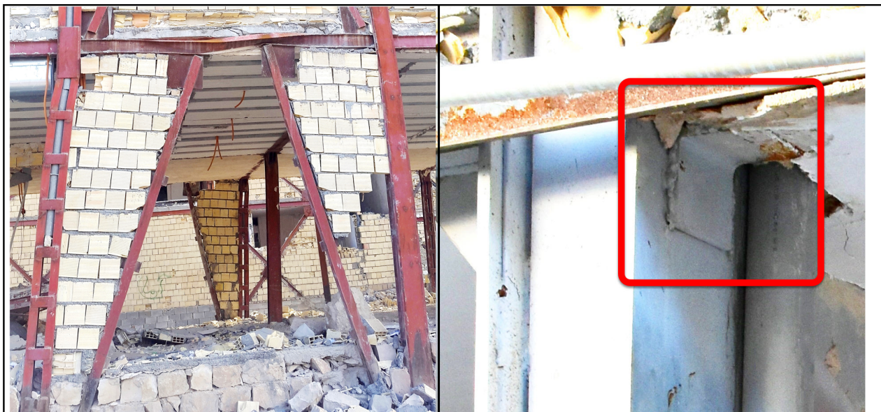
(a) Damage to beams which had no stiffener
