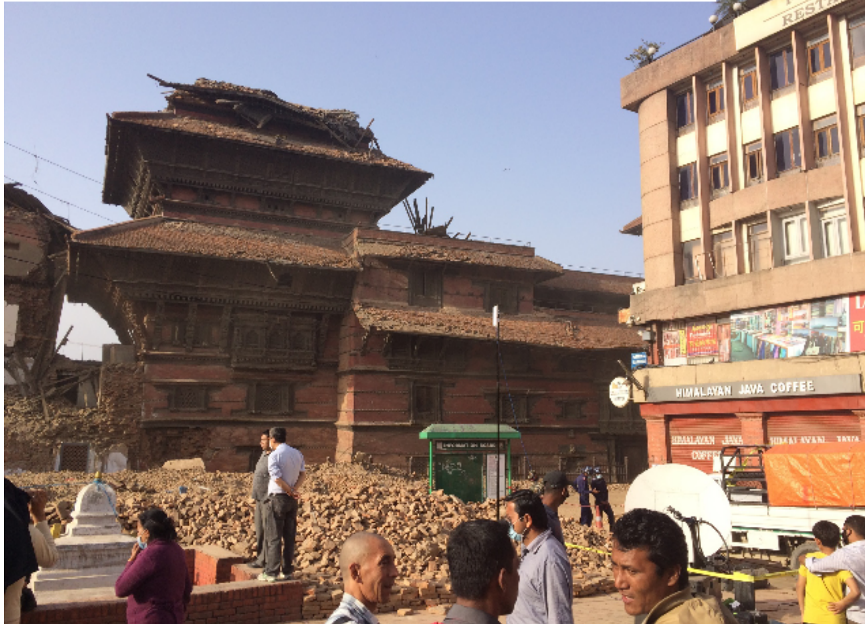
Heritage building collapsed but no damage to nearby RC building
