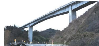
(a) Overall view
