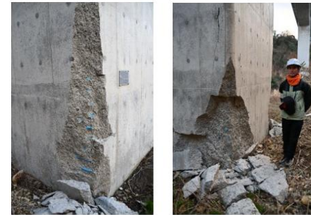
(b) Damage with spalling of concrete and exposure of rebar at the base of pier
