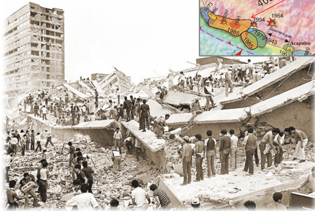
Nuevo León building, Tlatelolco, Mexico city
