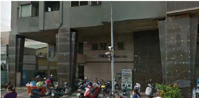
Southern Taiwan Earthquake of February 6, 2016
