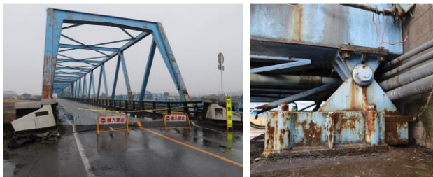
(a) West Side of Date Bridge.
