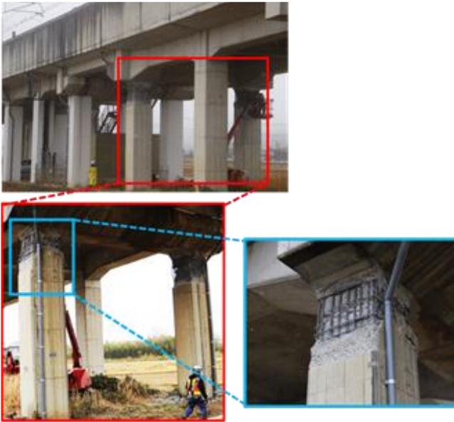
Photo 8 Flexure damage of RC pier in Shiroishi City, Miyagi Prefecture.(37°59'13"N, 140°37'33"E)
