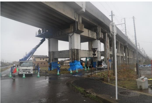
Photo 8 Flexure damage of RC pier in Shiroishi City, Miyagi Prefecture.(37°59'13"N, 140°37'33"E)
