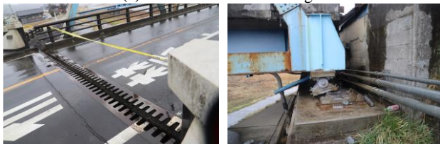
(b) East Side of Date Bridge.
