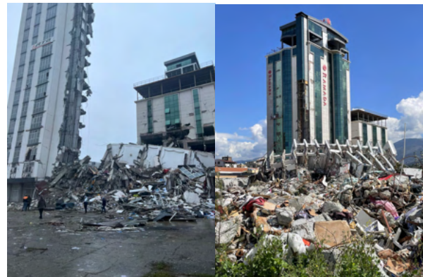
Fig. 13 A collapsed structure in front of Ramada hotel in Iskenderun (36.58899N, 36.17712E), photo on the left taken after first earthquake 17 ), photo on the right during the survey.
