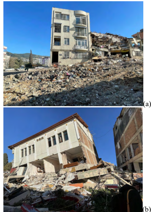
Fig. 17 Heavily damaged buildings in Antakya; (a) 36.19846N, 36.15393E (b) 36.20186N, 36.16133E.
