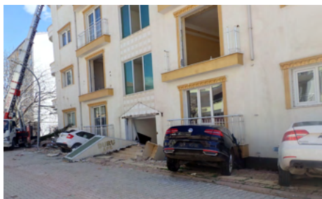
Fig. 4 Parked cars crashed under the settled building (37.787861N, 37.643083E).
