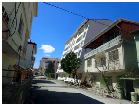
Fig. 3 Tilted houses in Golbasi, Adiyaman due to effect of liquefaction (37.787739N, 37.643769E).
