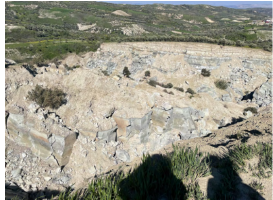
Fig. 19 A close up of top part of Tepehan landslide (36.1609N, 36.2211E)
