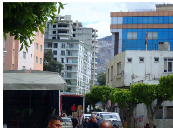
Fig.15 An example of tilted buildings in Cay Neighborhood, Iskenderun (36.587222N, 36.176639E).
