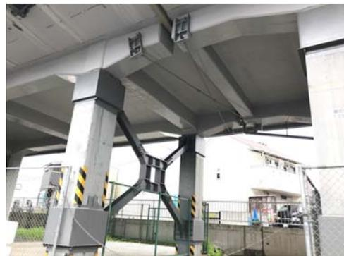
Fig.32 Situation of Tokaido Shinkansen Seismic Retrofitting (taken on June 19, 2018)
