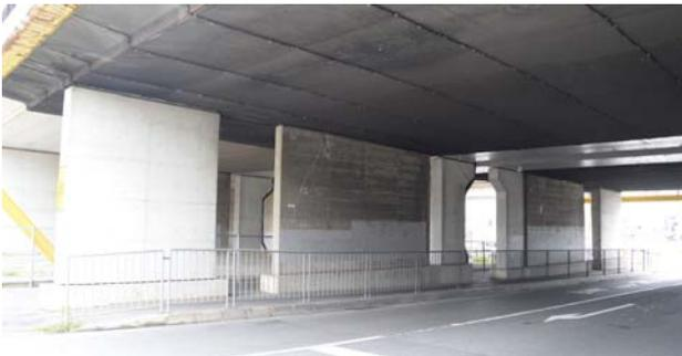
**Fig.34** Rocker pier added to both sides of the original intermediate piers at the widened part (taken on June 21, 2018)
