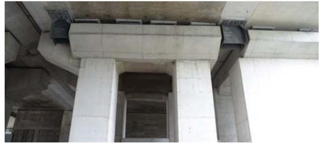
**Fig.35** Seismic retrofitting of rigid frame pier (taken on June 19, 2018)
