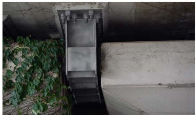
**Fig.37** Collision of stopper in transversal direction (taken on June 21, 2018)
