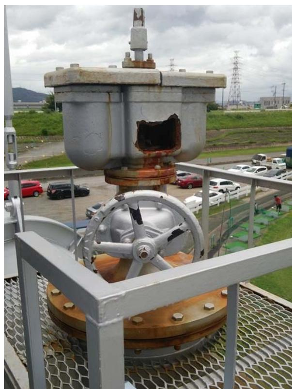
**Fig.20** Air valve of the Hirakata Water Bridge showing brittle failure of the air valve box
