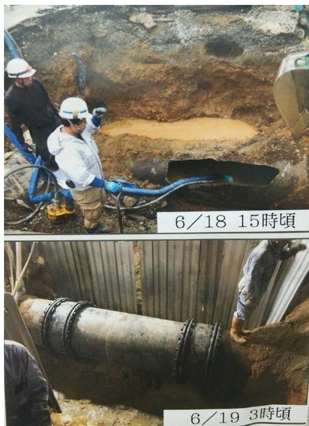
**Fig.17** Damage of water transmission pipe DIP (A) ( $\phi 900$ ) in Takatsuki City (from OWSA)
