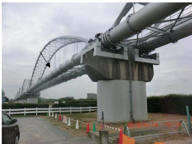
**Fig.19** State of Hirakata Water Bridge. Front 5 expansion line and rear side 4 expansion line. One of the leaked air valves is indicated by an arrow
