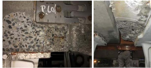
**Fig.27** Concrete failure at the joint of the PC rail girder (from Osaka Monorail)
