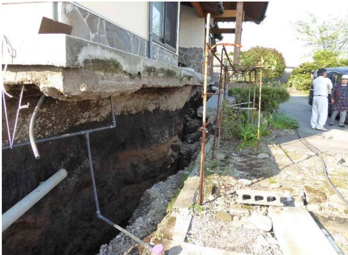
Fig. 3 House hanging a little over the northwestern offset of the ground at N32.9568°, E131.0368 (near Location No. 1)
