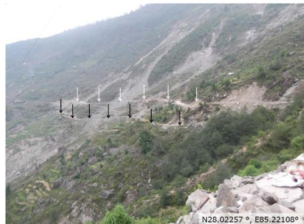
Fig. 10 Creeping section of Pasang Lhamu Highway: Black and white arrows show that the road constructed in 2003 (black arrows) has carried over about 30m horizontal distance from its original location (white arrows).
