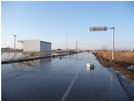
Photo 19 Broken wire fence of container terminal in Kashima Port, Photo courtesy of Ibaraki Prefectural Office
