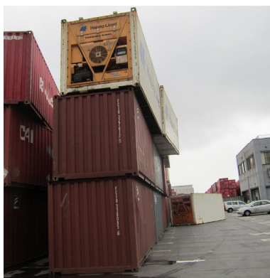
Photo 7 Displacement and Fallen Container in Triple stack due to the seismic effect,
