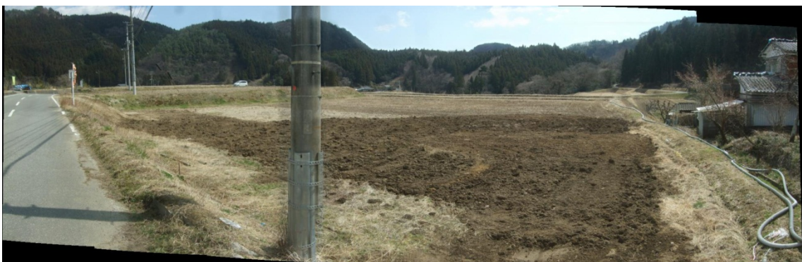
Fig. 3 Sinkhole (3m × 7m × 1.5m deep) at Tabito plugged up (Photo by Kazuo Konagai at 36.951532, 140.700233 on March 27 th , 2012).
