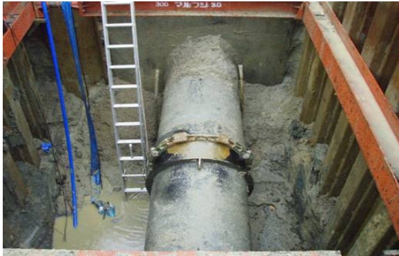
Photo 2 Excavation of joint failure portion.
