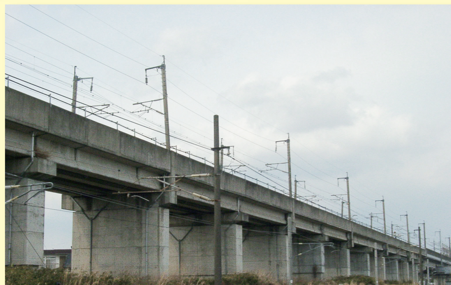
The Tohoku Shinkansen elevated bridge (Fukushima Prefecture) had only minor damage.
