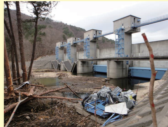
The Fudai floodgate (Iwate Prefecture) prevented tsunami runup.
