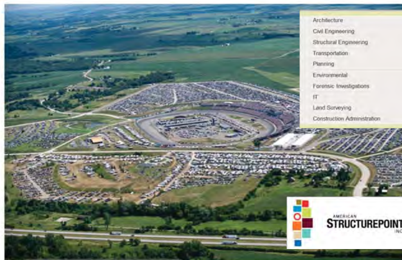
Completed $70-million Iowa Speedway. Image courtesy of American Structurepoint, Inc.
