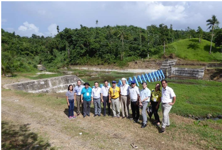
Slit Dam in Ormoc City, Leyte Island, the Philippines
