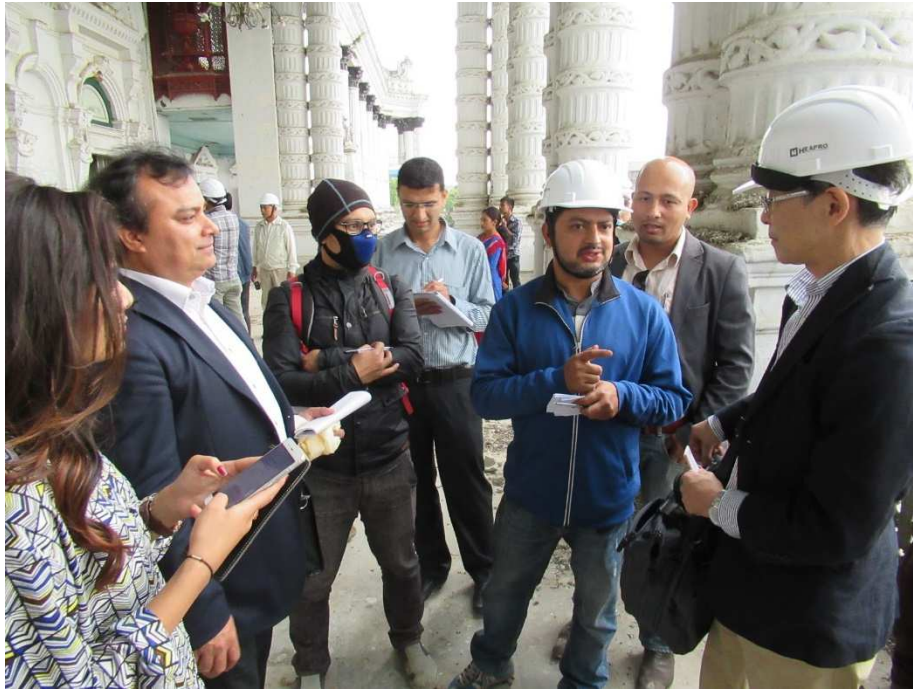
Historical Former Prime Minister's Office building in Kathmandu damaged by 2015 Nepal Earthquake
