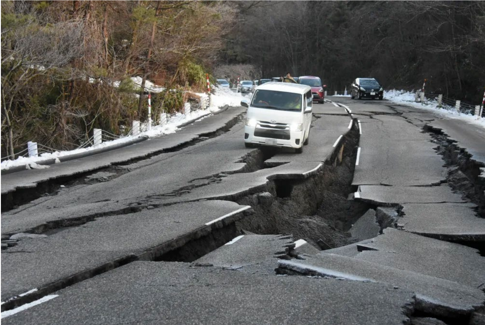
A buckled road caused by the Jan. 1 earthquake in Noto, Ishikawa Prefecture
