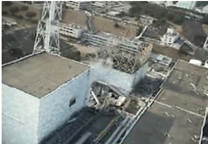
Fukushima Daiichi Nuclear Power Station
