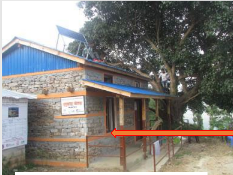
Wooden seismic Beam/Band
