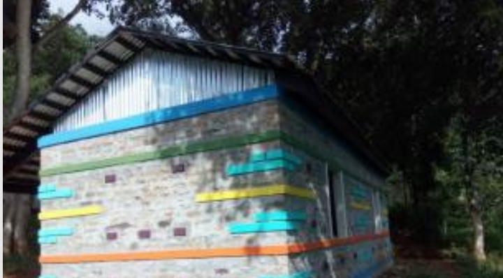
Model building showing earthquake resilient elements at community
