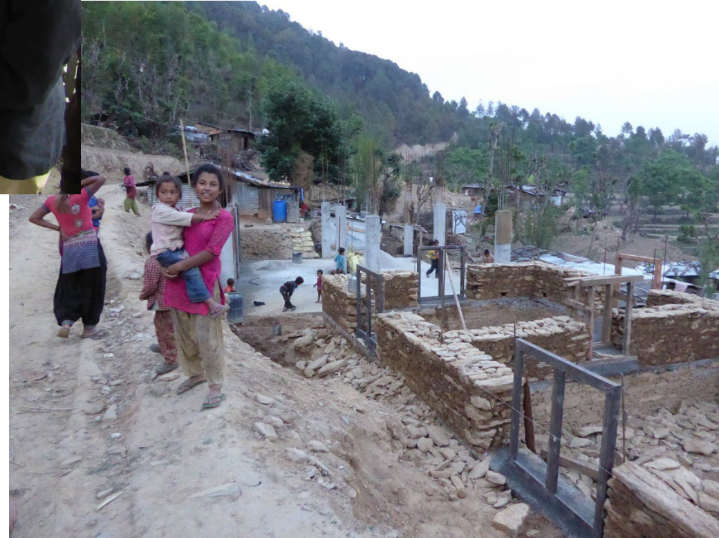
Reconstruction works of housings in Irkhu Village, Sindhupalchowk District
