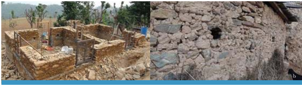
Photo 3 Reconstruction works of housings being performed in Irkhu Village, Sindhupalchowk District. (a) Housing under construction, showing the horizontal concrete reinforcement (band) placed between stone layers in contrast to the old warehouse without the horizontal reinforcement (b).
