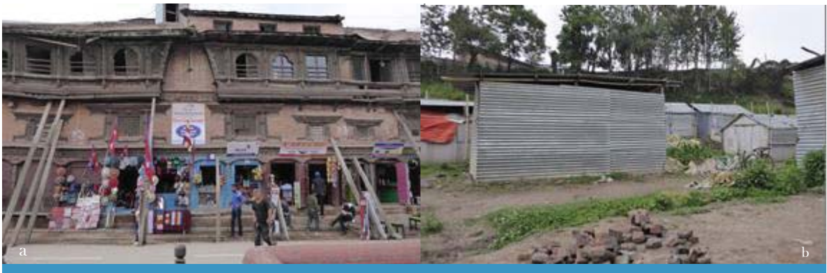
Photo 4 A number of historical buildings are being reconstructed in the ancient city, Bhaktapur. The left photo shows a building supported by timbers for anti-earthquake purpose. The right photo shows the temporary housings for the 2015 earthquake victims.
