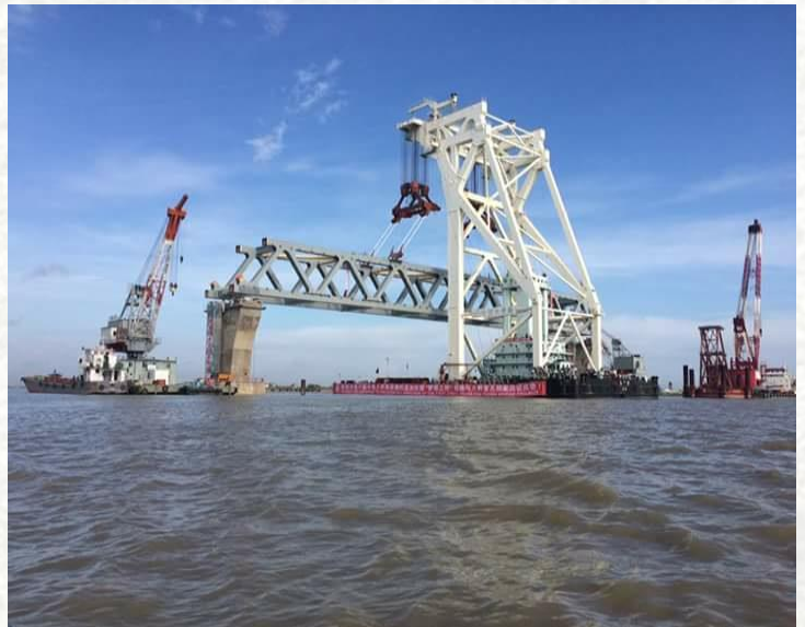
First Span Installation on the Pier 37 & 38
