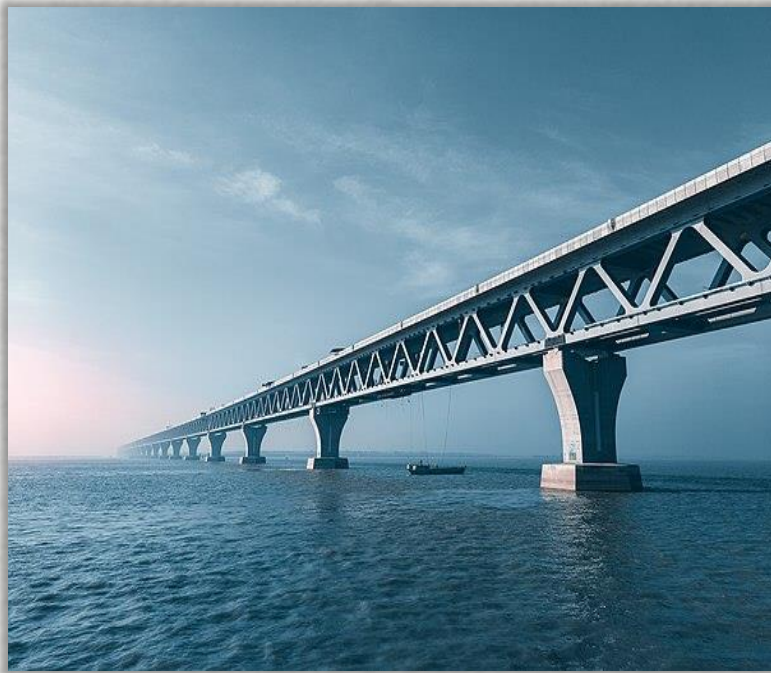
Padma Bridge in November, 2021
