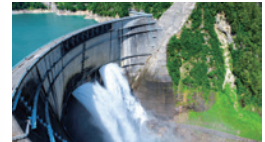
Kurobe No. 4 Dam
