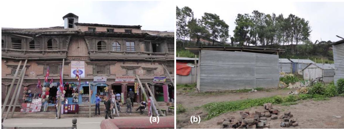
Photo 4 A number of historical buildings are being reconstructed in the ancient city, Bhaktapur. The left photo shows a building supported by timbers for anti-earthquake purpose. The right photo shows the temporary housings for the 2015 earthquake victims.
