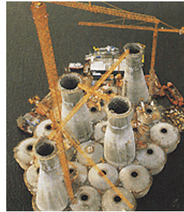
Condeep (abbr. concrete deep water structure )
