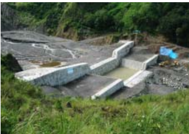
Fig. 9 Upstream view of concrete Sabo Dam No 7-3 in Jeneberang River (photograph by Hazama, 2007).
