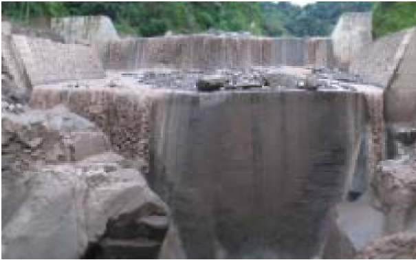
Fig. 7 Downstream view of concrete Sabo Dam No 7-1 in Jeneberang River, 7 km far from Mt. Bawakaraeng (photograph by Hazama, 2007).
