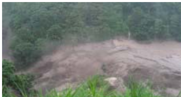
Before debris-flow(upper), During debris-flow(lower) Fig. 4 Sabo Dam No.7-1 before and during debris-flow (event with this debris-flow is only one, since series of Sabo Dams have been constructed).
