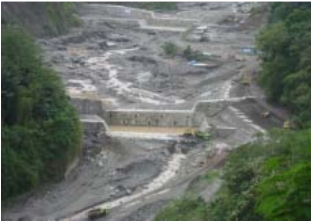
Fig. 8 Downstream view of concrete Sabo Dam No 7-2 in Jeneberang River (photograph by Hazama, 2007).
