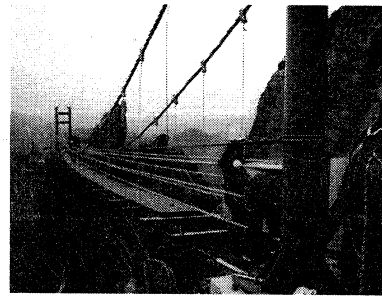
Figure 20. Installation of snap-fit composite deck for a pedestrian bridge
