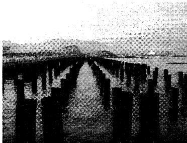
Figure 16. Pile foundation of Noolcha Bridge before installation of decks
